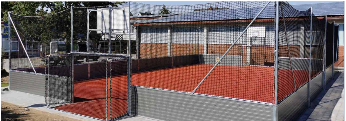
SoccerGround Multisport, Dörentrup, 65' × 42'
