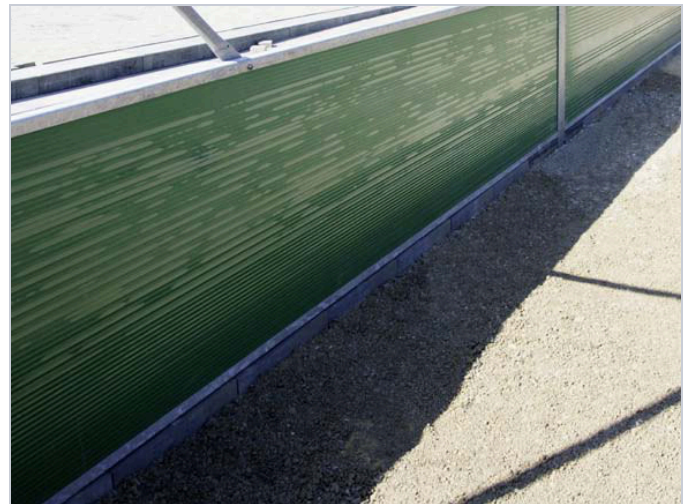
Like this. Curb placed correctly (inner edge flush with boards).
