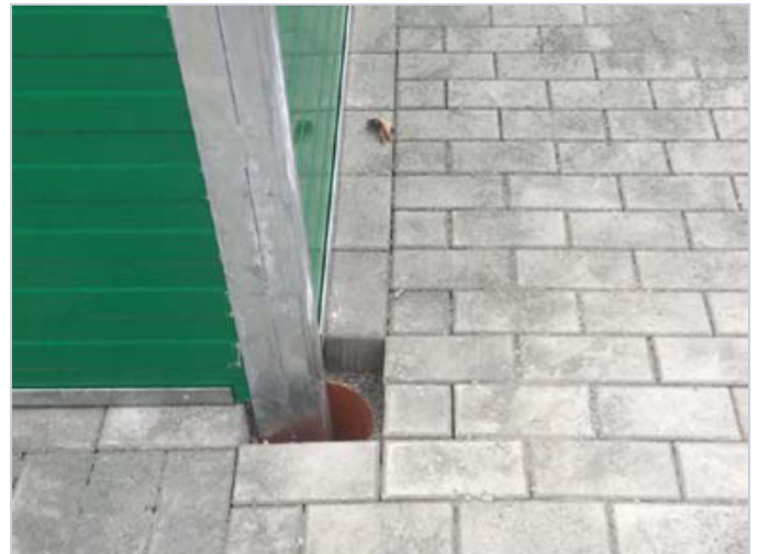
Like this. Curb built right up to the conduit; paving can be laid up to it after filling.
