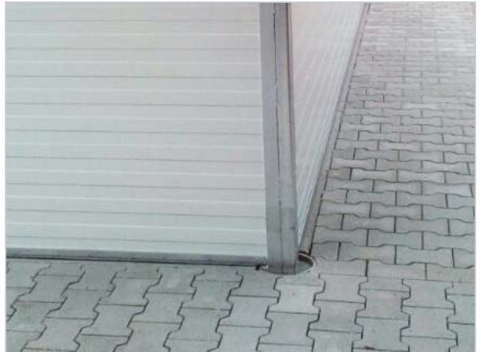
Like this. Foundations / conduits placed per foundation plan.
