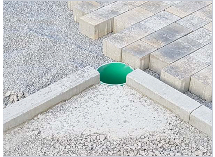
Like this. Accessible conduits, closed with lids if necessary, ideally ending at the top of the gravel.
