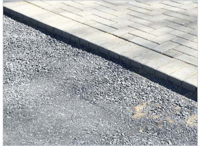
Like this. Even installation height, as specified.
