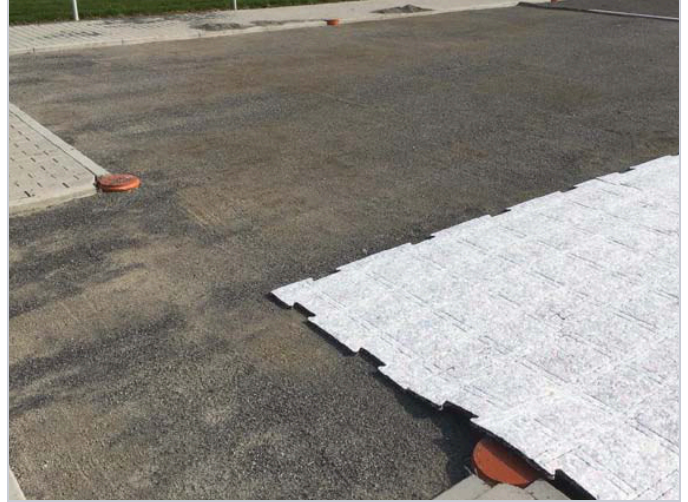
Like this. Gravel leveled and firmly compacted.
