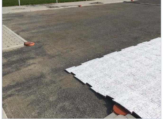
Like this. Gravel leveled and firmly compacted.
