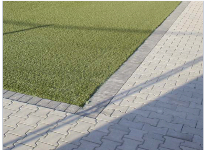
Like this. Surrounding paving level.
