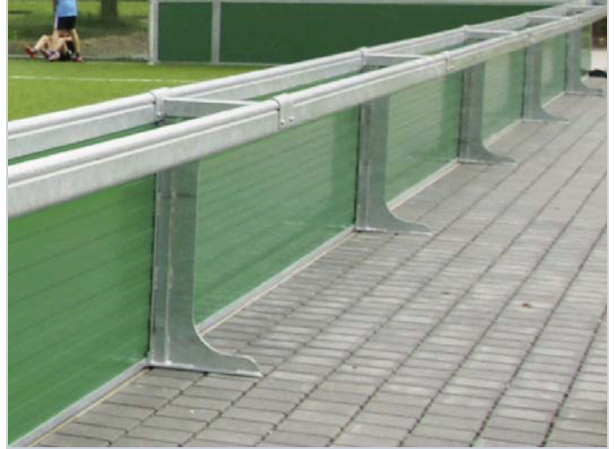
Like this. Curb and paving level, so the feet stand flat.
