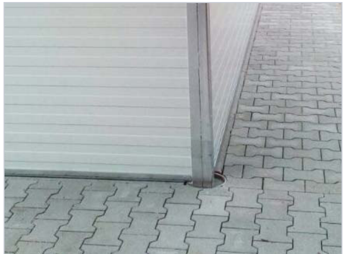
Like this. Foundations placed per foundation plan.
