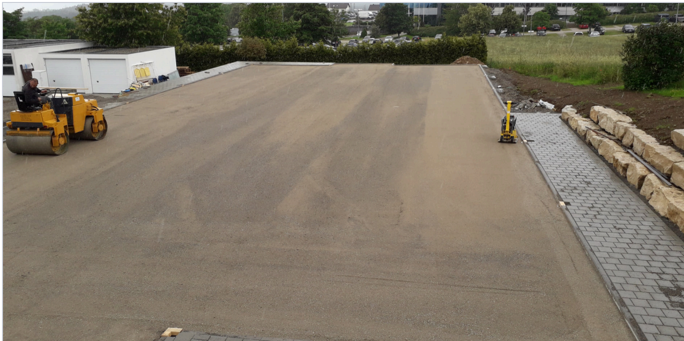
Gravel layer level and evenly compacted, firm and shear-resistant
