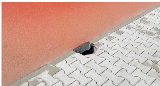
Installed artificial turf
