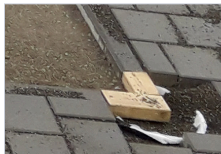
Corner post foundation formwork
