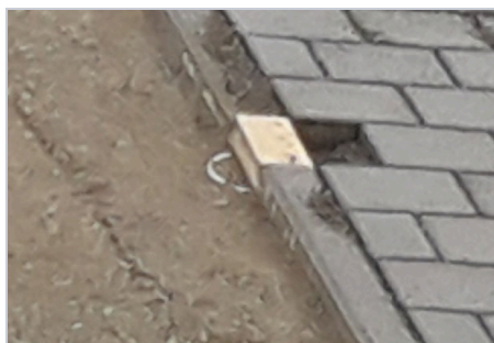
Side post foundation formwork
