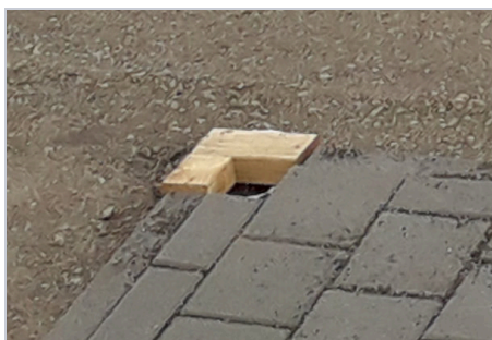
Goal post foundation formwork
