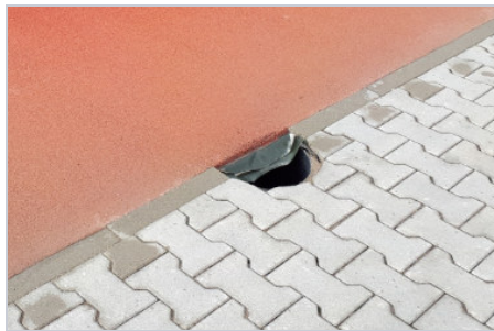
Court inside · installed artificial turf
